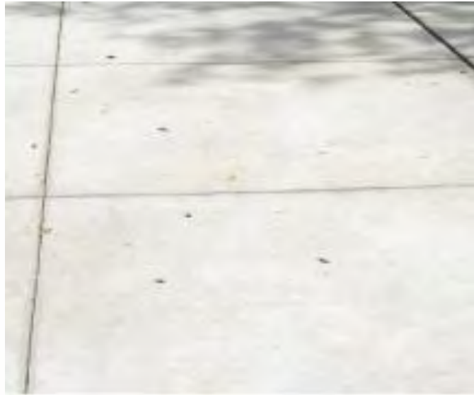
Medium Broom Finish Concrete
