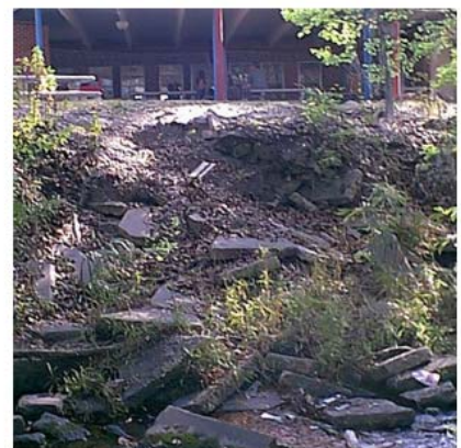
Tumblin Creek bank failure at PK Yonge Developmental School
