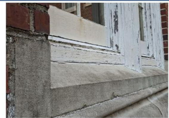
Fig. 4.16. Staining and some mold growth on cast elements and mortar joints. Photograph: Walker Architects, 2025.
