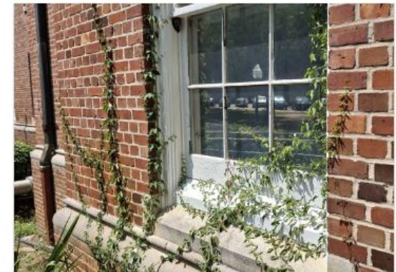
Fig. 4.20. Example of area in shade and/or near condensate drains with excessive plant growth. Photograph: Walker Architects, 2025.
