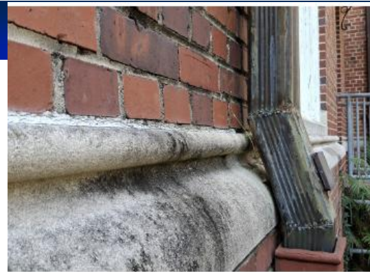
Fig. 4.15. Staining and some mold growth on cast elements and mortar joints. Photograph: Walker Architects, 2025.
