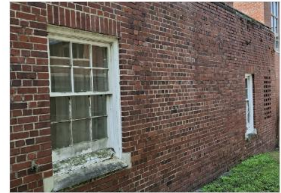
Fig. 4.18. Example of brick staining and mold growth. Photograph: Walker Architects, 2025.
