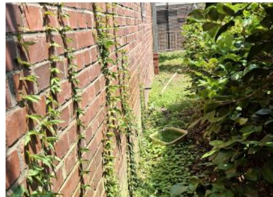
Fig. 4.19. Example of area in shade and/or near condensate drains with excessive plant growth. Photograph: Walker Architects, 2025.
