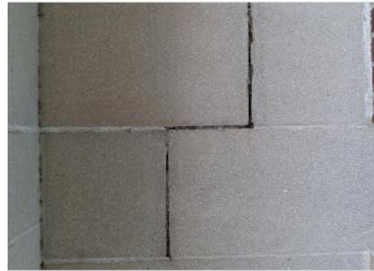
Fig. 4.17. Example of mortar in need of repair. Photograph: Walker Architects, 2025.
